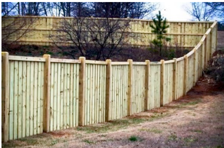
Figure 25-5.5.6: Fence with Finished Side Out
