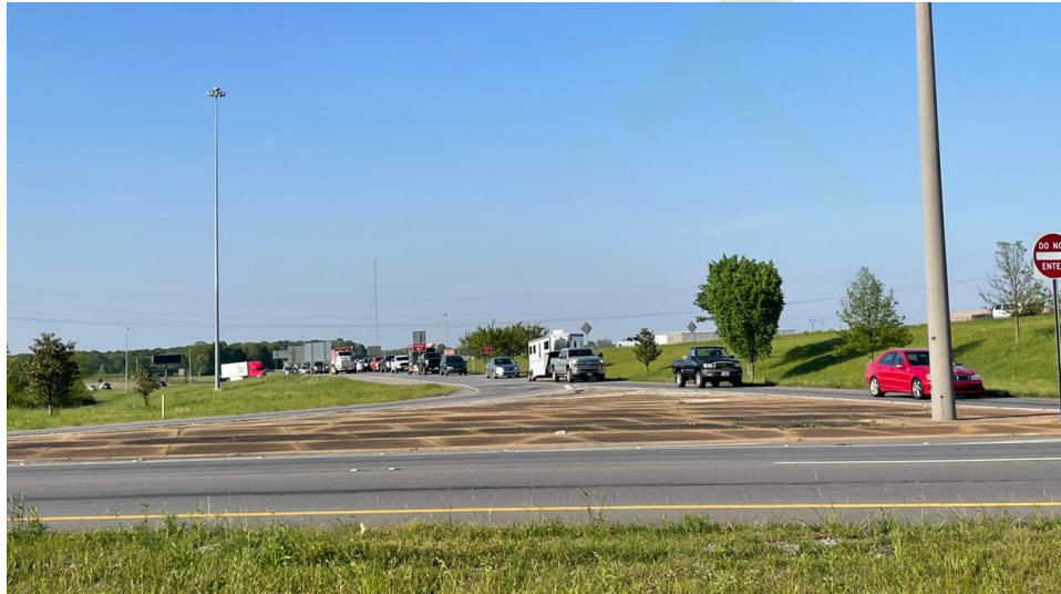
Figure 2: Southbound Approach at I-65 SB Ramps/SR 67 Intersection
