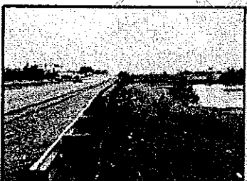
4 Some areas will require special thought as embankments are not wide enough for the Bikeway.
