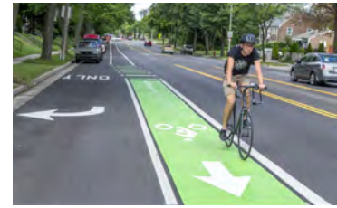
Painting bike lanes green is one way to promote awareness of the trail system's on-street facilities and improve safety.
