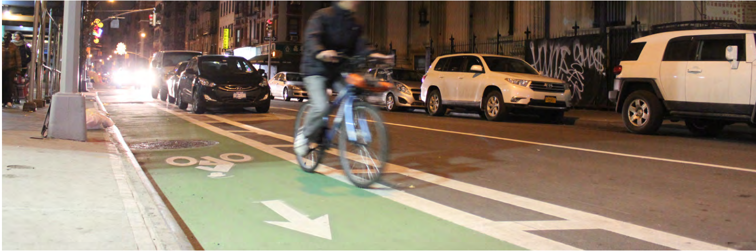
Street Level Separated Bicycle Lanes can be separated from the street with parking, planters, bollards, or other design elements.
