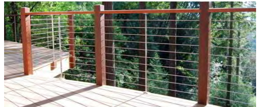
(Above) Cable railing with timber posts and handrail.
