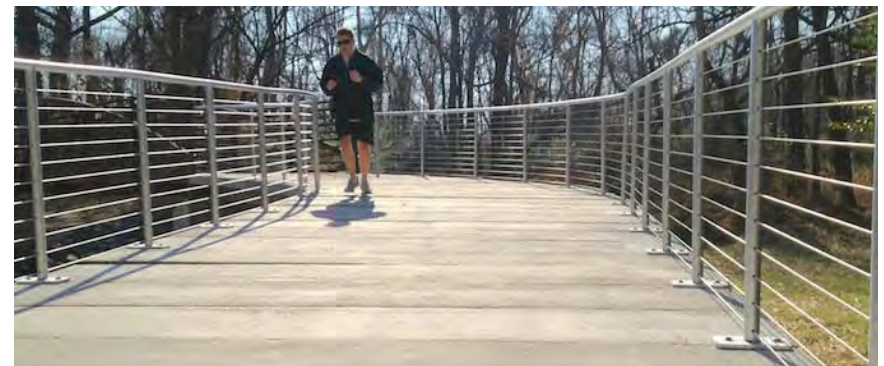
(Above) Cable railing with aluminum posts and handrail along boardwalk.
