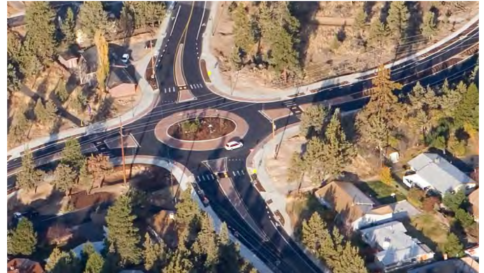
This roundabout features designated ramps that transition people on bicycles from the bike lane on to a shared use path or wide sidewalk. People on bikes are then directed back on to the roadway, or across a marked crosswalk. Crossings are set back from the circulatory lane and orient people walking and on bikes so that they are better able to see oncoming cars.
