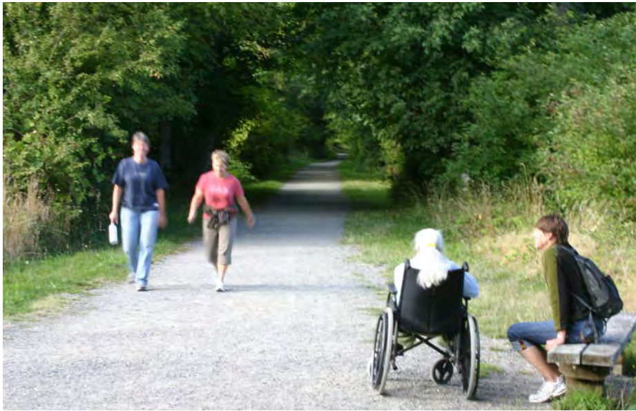
(Above) Some gravel and crushed fine material trail types are considered to be ADA-compliant. Source: National Trails Training Partnership
