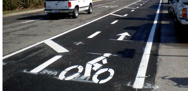
The use of pavement markings delineates space for cyclists to ride in a comfortable facility.
