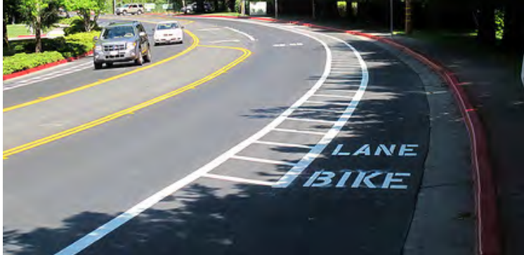
The use of pavement markings delineates space for cyclists to ride in a comfortable facility.
